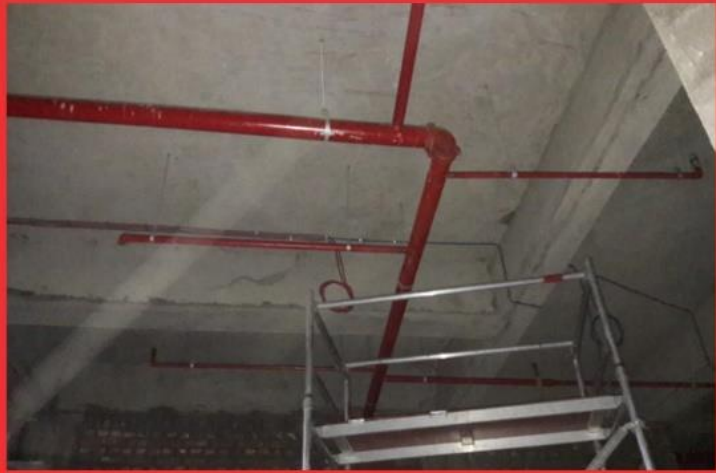
SPRINKLER PIPING WORK
