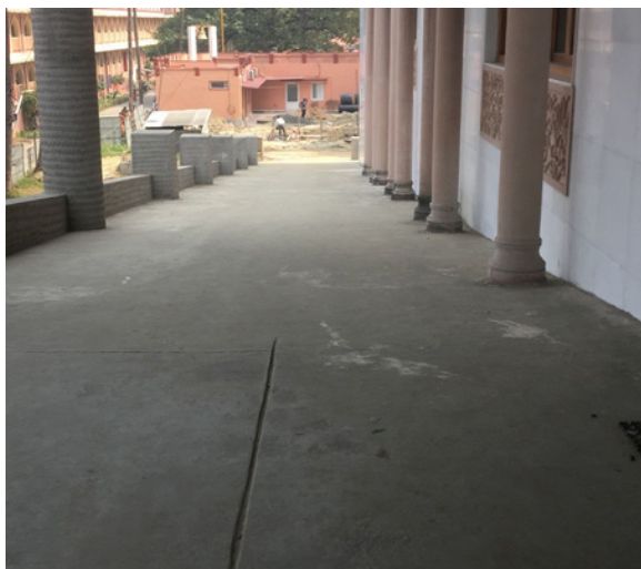
Rear Ramp Flooring
